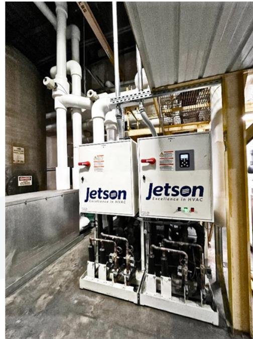
Designed for easy retrofit - fits through a standard three-foot door and can be serviceable from the front of the unit.
